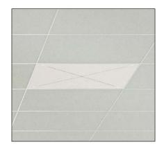
Variant 1 installed flush in a dropped/coffered ceiling (600 x 600 mm)
